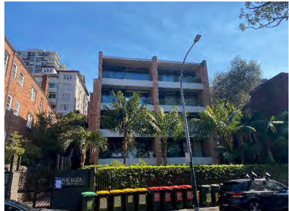
Figure 4.11 The brick fins of the side elevations are expressed by the generous separation walls between apartments. Balustrades are fitted to the concrete spandrels.
